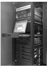
Front of a rack
